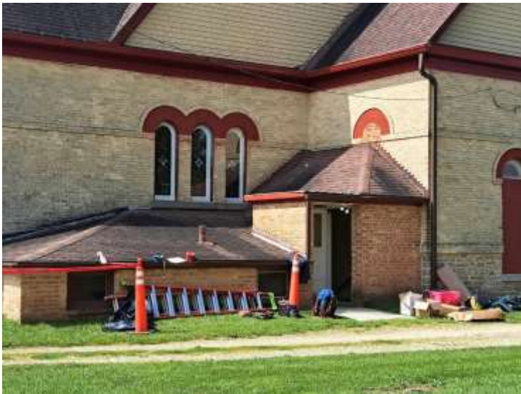
Barrier free construction has started on the Upper Church!
